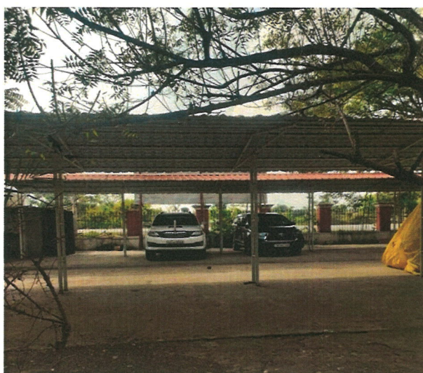
Figure 12. Roofed Parking for Four Wheeler's
